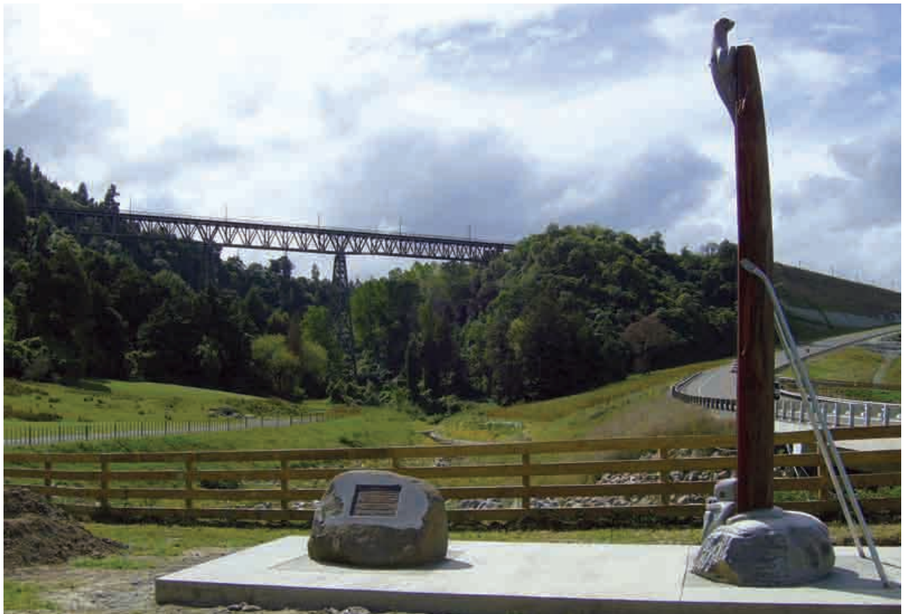
The plaque unveiled by IPENZ recognises the engineering heritage of Makohine Viaduct. The Heritage Board promotes items of engineering significance such as the viaduct, which at its completion in 1902 was thought to be the second highest in the world. Image courtesy of Mike Mellor.
